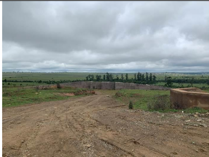
Figure 18: Dutywa waste transfer station entrance
