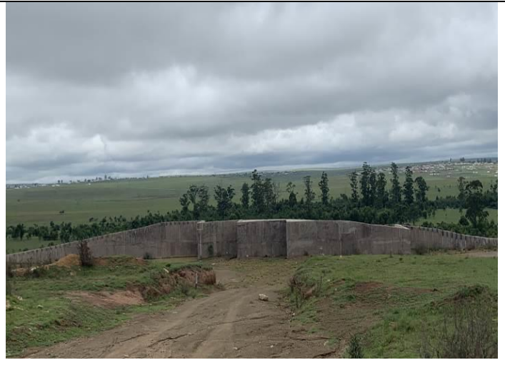
Figure 19: Current infrastructure of the non-operational transfer station
